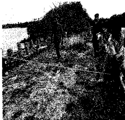
Fig.4. Narrow stretch of coconut piled bund (1.5 m) at the eastern side.
