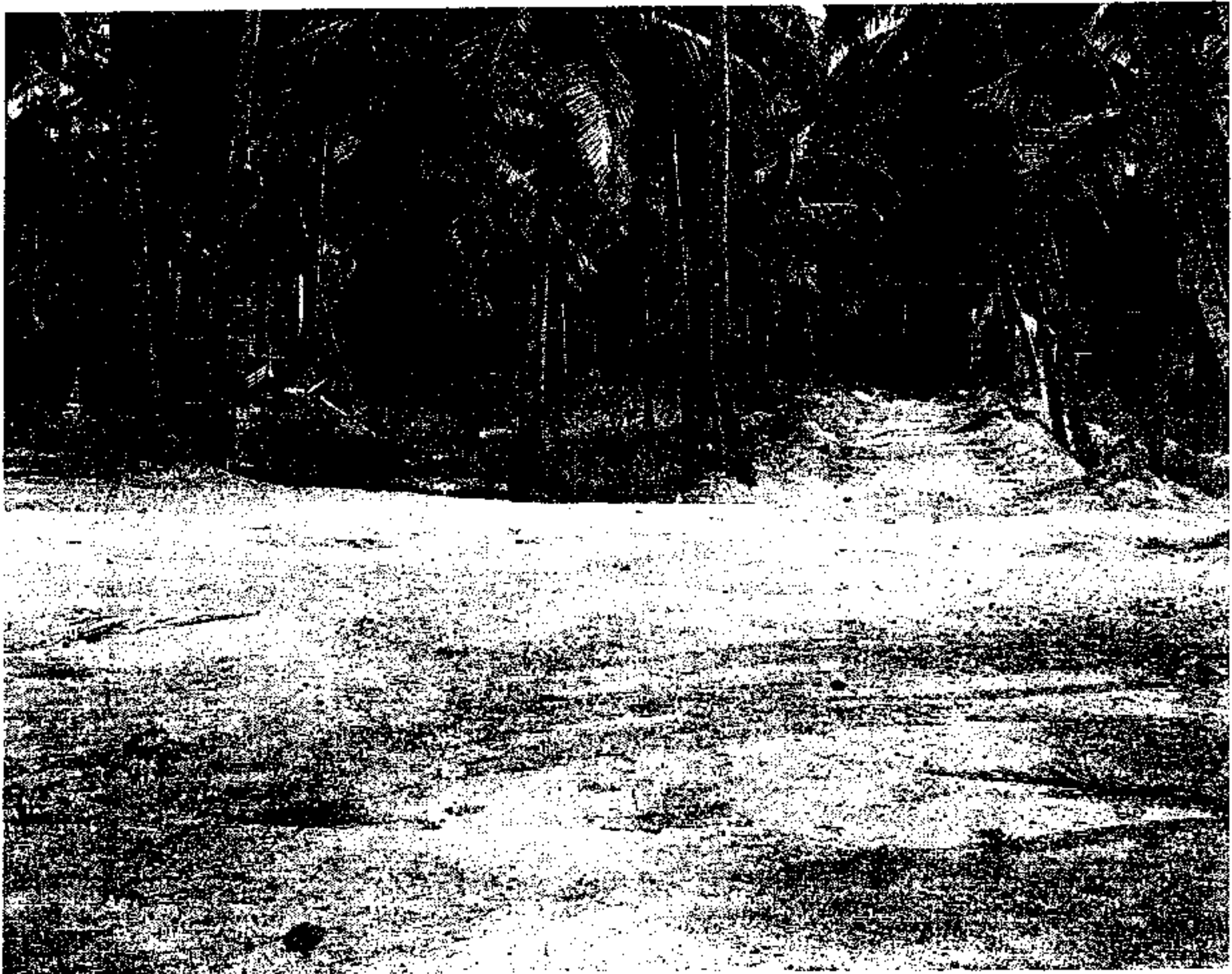
Plate 2: Reclaimed area and the construction of Hotel
