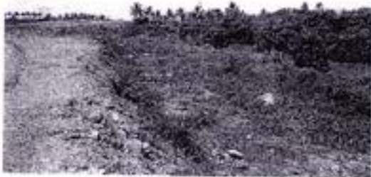
Fig 3. Road & Reclamation blocking flow of tidal water to mangroves along the road towards LNG Storage/ terminal from Vypin (Goshree Jn)
