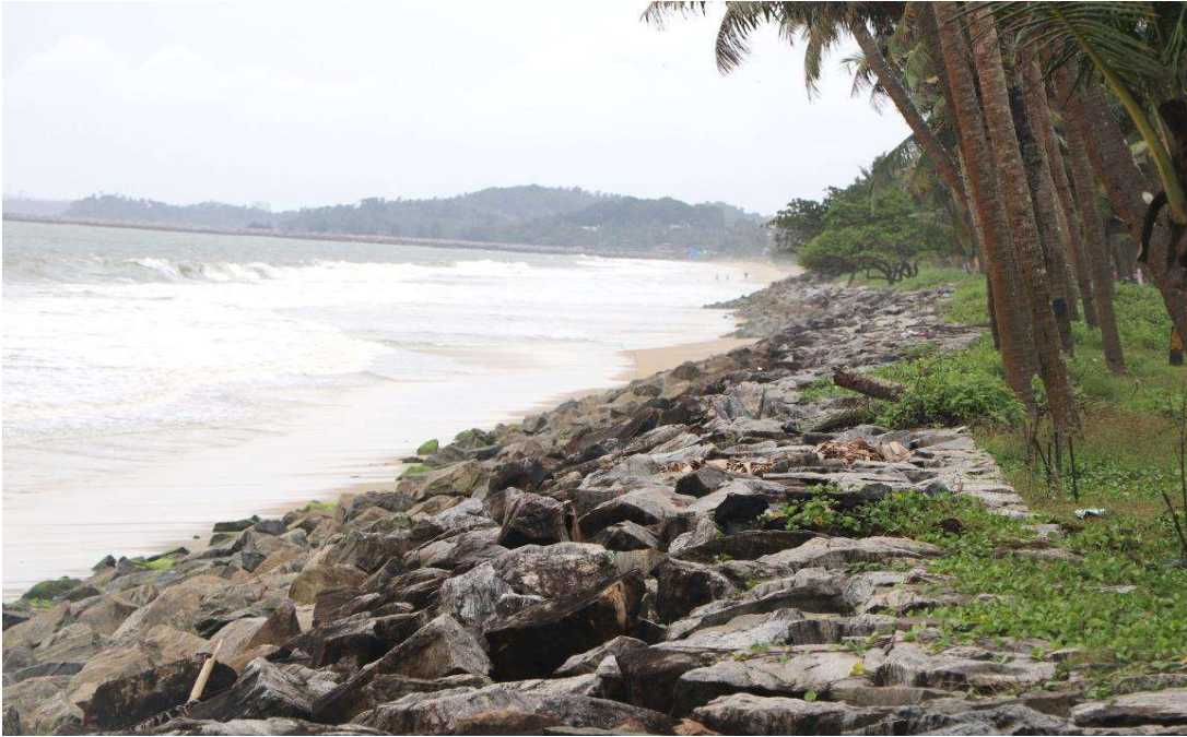
Plate-3: HTL at Thayyil Beach (Location: 75° 32' 46.51" E 11° 40' 25.11" N, Azhiyur Panchayat, Village: Azhiyur)
