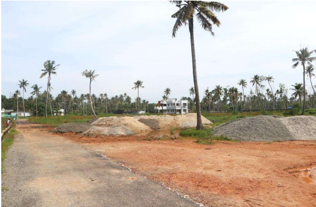
Plate-5: Mangrove area found to be removed at Neelashwaram thoppu, Thuruthu (Location: 76° 32' 55.19" E 8° 56' 35.48"N, Neendakara Panchayat, Village: Neendakara)
