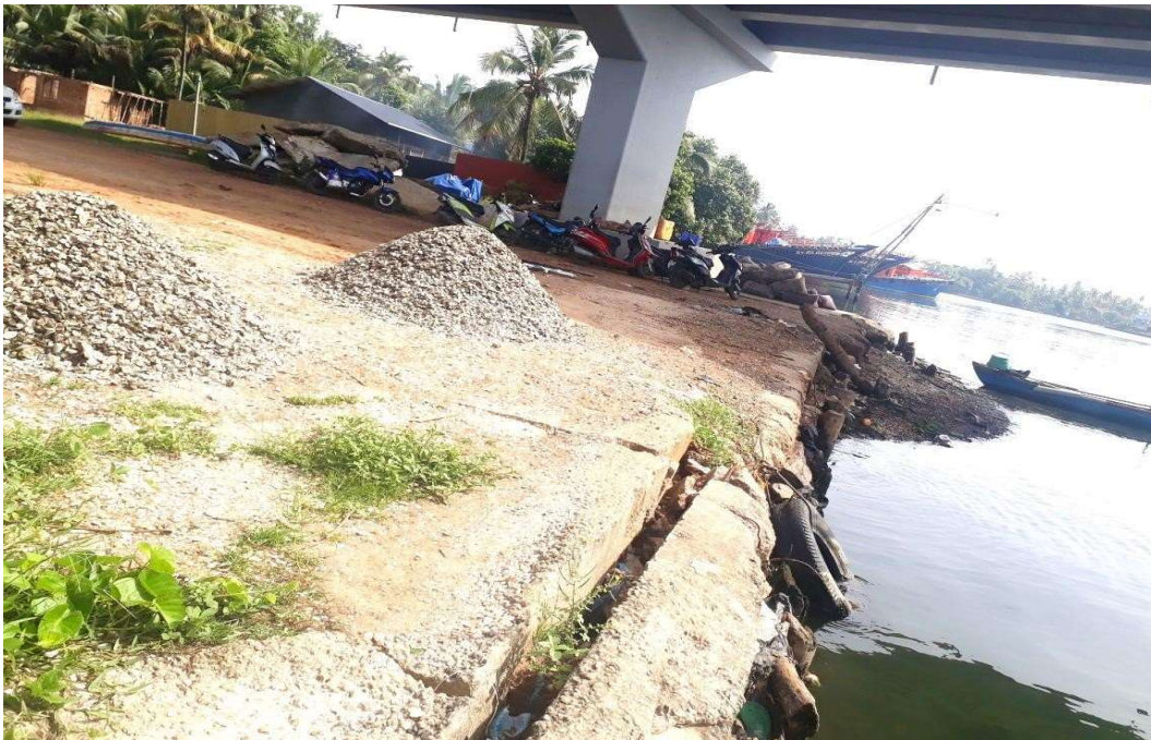
Plate 10: Mangrove area found to be removed at Kavanad bridge (Location: 76°33'43.24"E 8°55'24.75", Kollam Corporation, Village: Thrikkadavoor)
