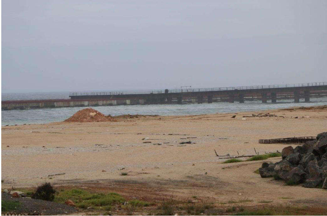
Plate-1: HTL at Vizhinjam Port (Location: 76° 59' 46.60" E 8° 22' 23.13" N, Thiruvananthapuram Municipal Corporation, Village: Vizhinjam)
