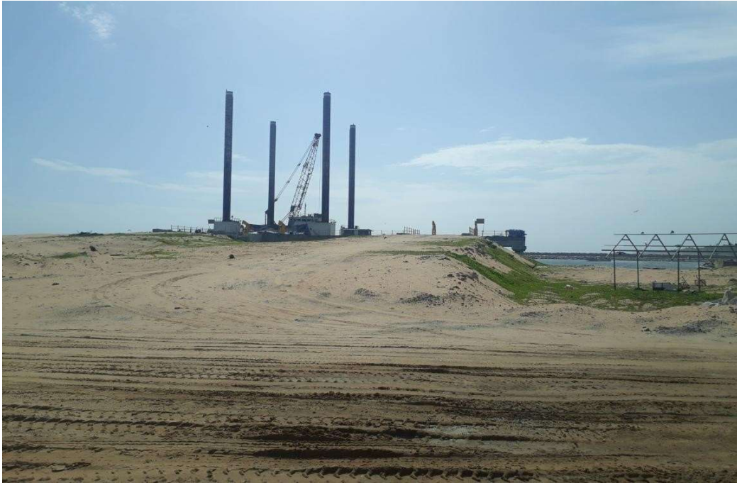
Plate-7: HTL at Perumathura harbour (Location: 76° 47' 14.99" E 8° 37' 55.06"N Chirayinkeezhu Panchayat, Village: Sarkara-Chirayinkeezhu)
